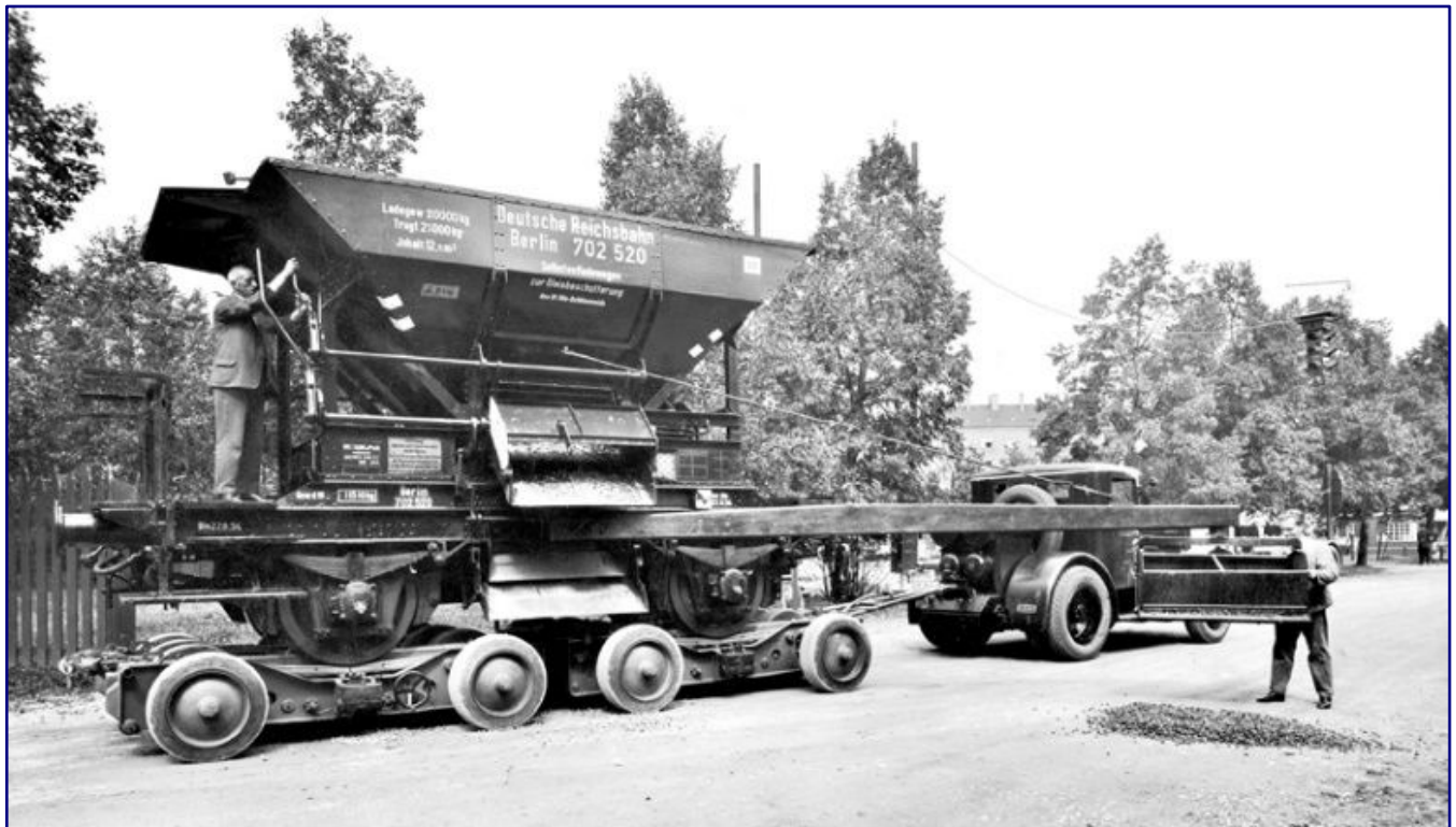
At a road construction exhibition held in Munich in 1934, the 20 t ballast wagon on a road roller demonstrates its basic suitability for road construction when filling in potholes. The Talbot-built self-unloading wagon for track ballasting "Berlin 702 520" is a real classic of railway service wagons. Photo: RVM, Eisenbahnstiftung
