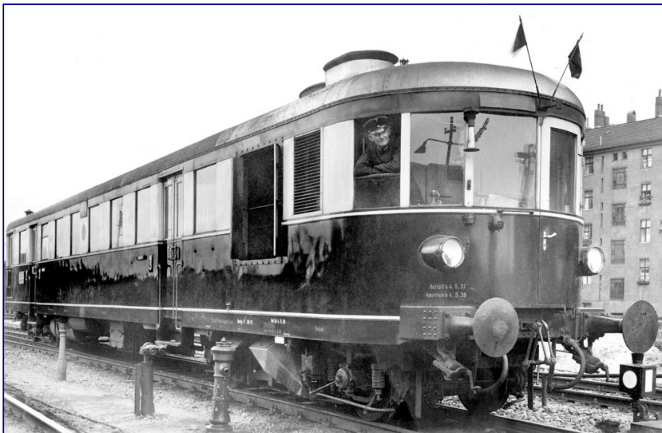
Influenced by the success of fully automatic steam generation systems, eight steam railcars (DT 51 to 58) were built by Borsig, Henschel and Wegmann for the Reichsbahn between 1934 and 1938. Hermann Maey had the new DT 53 driven into position in Berlin Stettiner Bahnhof on 4 May 1936. Photo: DLA Darmstadt (Hermann Maey), Sammlung Eisenbahnstiftung
